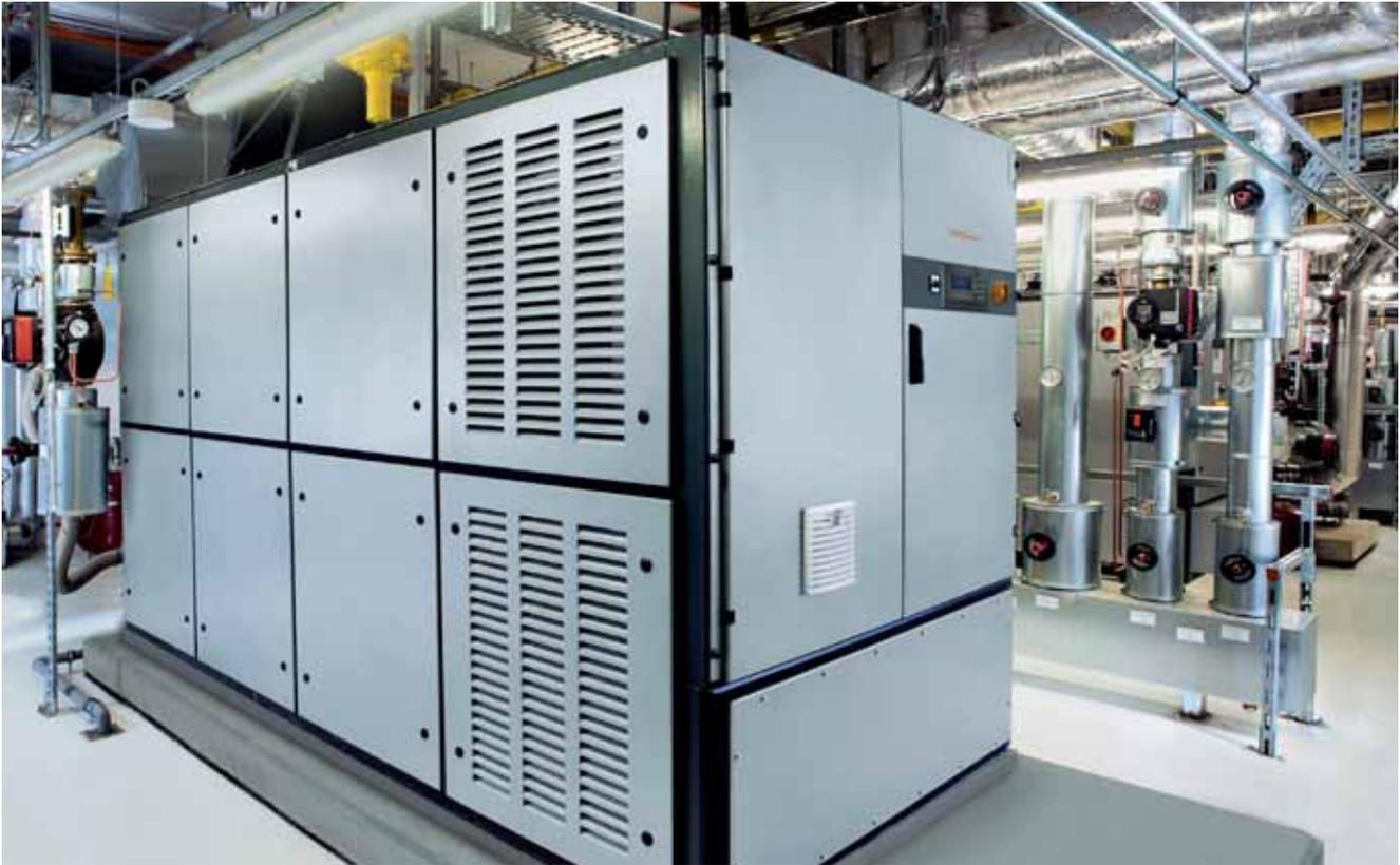
Viessmann CHP units achieve a total efficiency of up to 95 percent. Together with the simultaneous production of electricity and heat, this makes CHP units extremely efficient.
