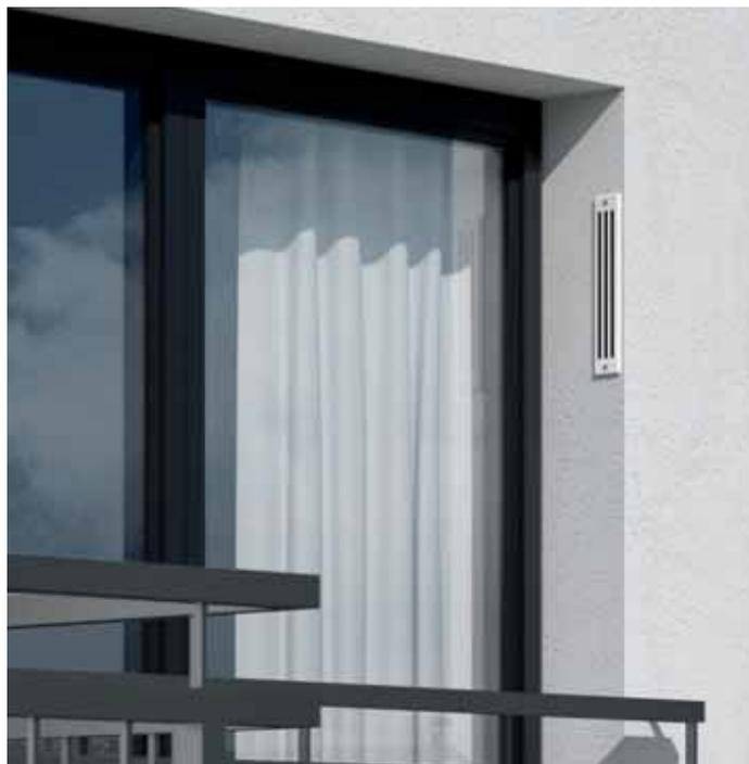
Unobtrusive appearance due to installation of the Vitovent 100-D in the window reveal
