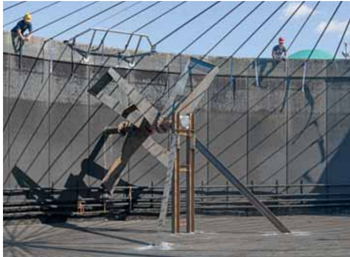
Installation of new, more powerful components
