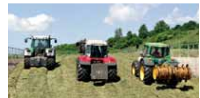
Compaction of the delivered regenerative raw materials
