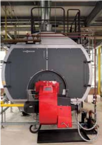
Viessmann steam and hot water generators are characterised by high efficiency.
