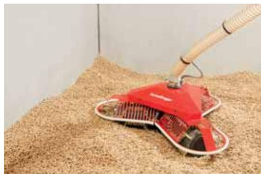
Storage room with supply to the pellet boiler via mole system
