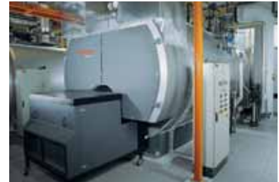
Vitomax RS steam boiler with waste heat utilisation and burner
