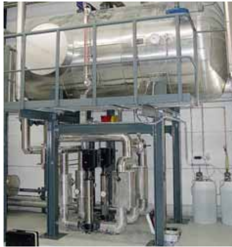
Pre-assembled feedwater pumps and tanks
